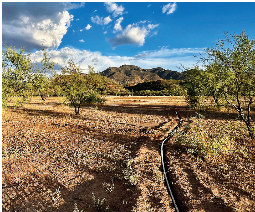
Irrigation lines are being laid among mesquite trees, with Red Mountain in the background. | Photo by Mary Tolena
