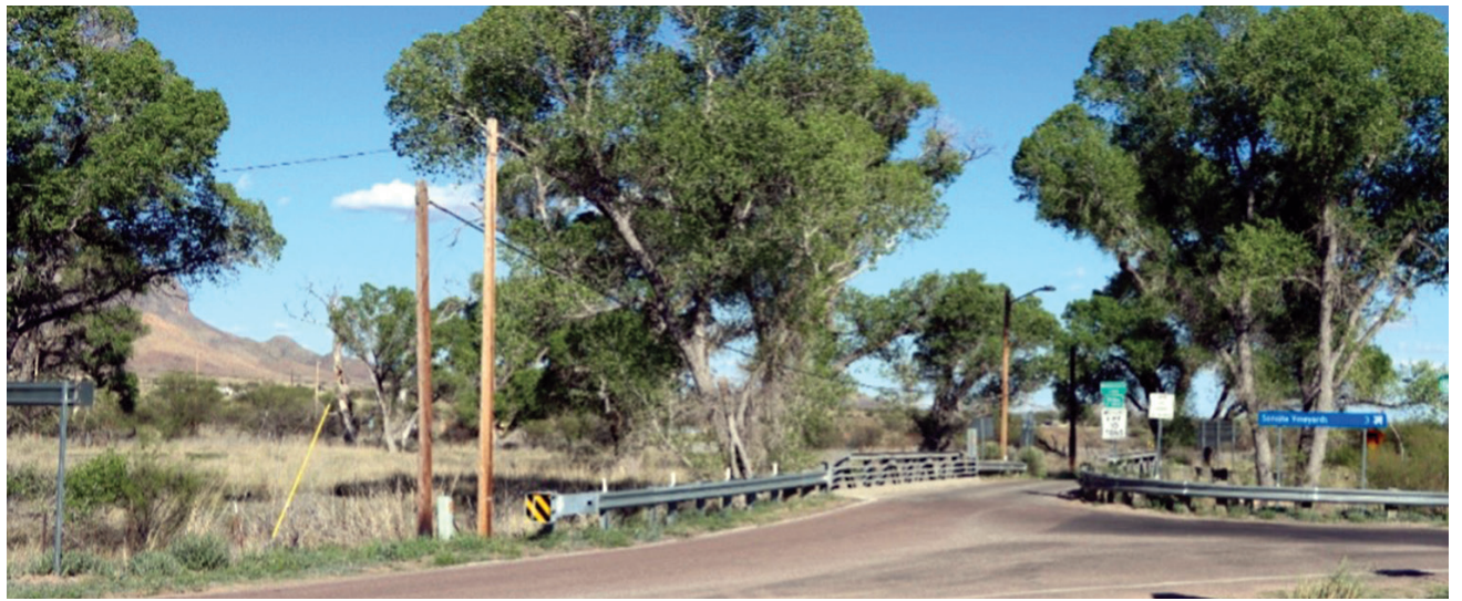
Guardrails on the Elgin Bridge today may be different, a result of work done by Tucson bridge engineer Jerry Cannon in 1999, but the structure of the bridge has not been altered. | Photo by Carrie White
